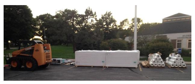
**Roof Insulation.** The stack of insulation in the middle of the picture, above, provided an additional 1" of insulation on the roof. This was a 25% increase.
